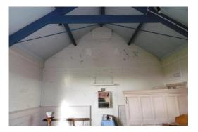
4.3.1 Description: The main space is divided into five bays, separated by 4no. trusses. There is an exposed ridge beam. One purlin is centrally located on each pitch.
